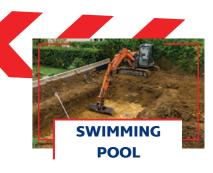
Digging to the exact dimensions and slope of the pool becomes child's play with the iDig guidance system.
