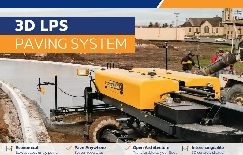
Ligchine International has partnered with Topcon Positioning Systems to offer the revolutionary '3D LPS' system (local positioning system) for Concrete Paving as a ScreedSaver option. The combination of Ligchine's boom operated ScreedSaver machines with Topcon's "LPS system" guarantee you the lowest cost entry point into 3D paving; amazing ease of use; significant labor savings; high volume production; and world class accuracy whether operating indoors or outdoors.
