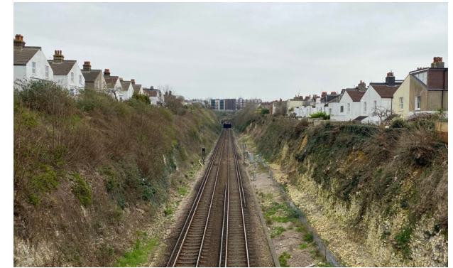
Picture 1: Typical cutting in southeast England
