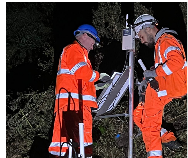
Picture 3 & 4: Installing InfraGuard in Wessex during a night-time shift
